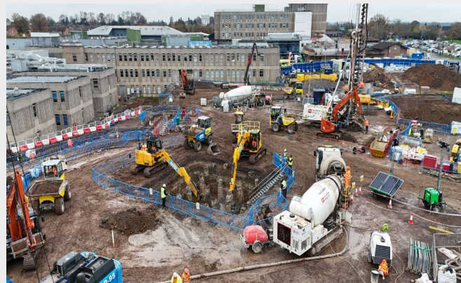
Piling work progress
