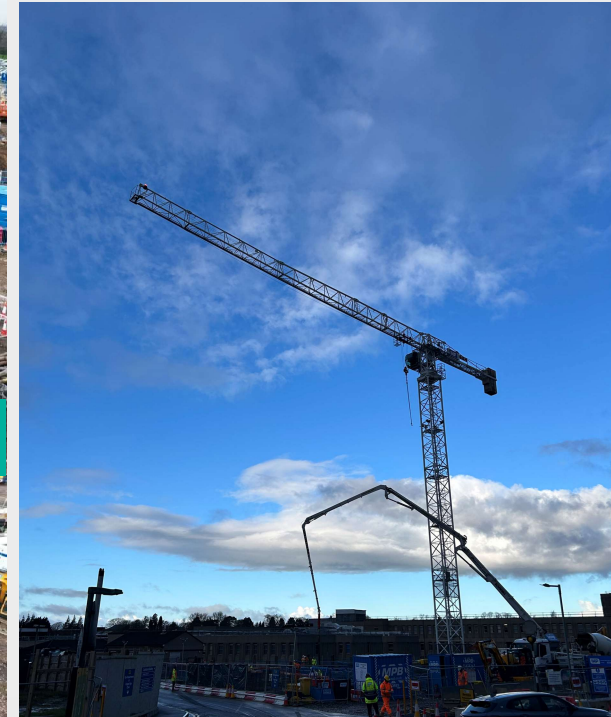
The first of two cranes has arrived on the construction site
