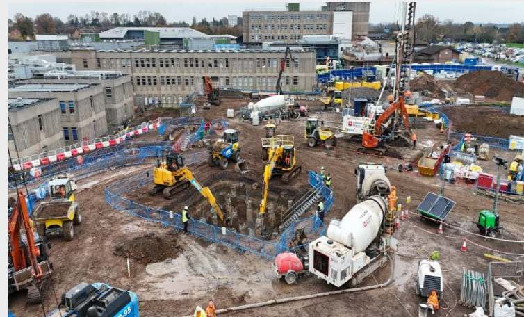
Piling work progress
