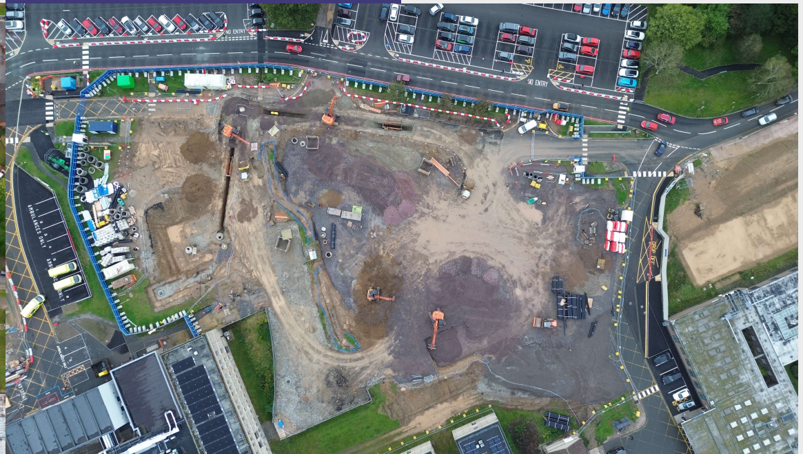
RSH site during site preparation works
