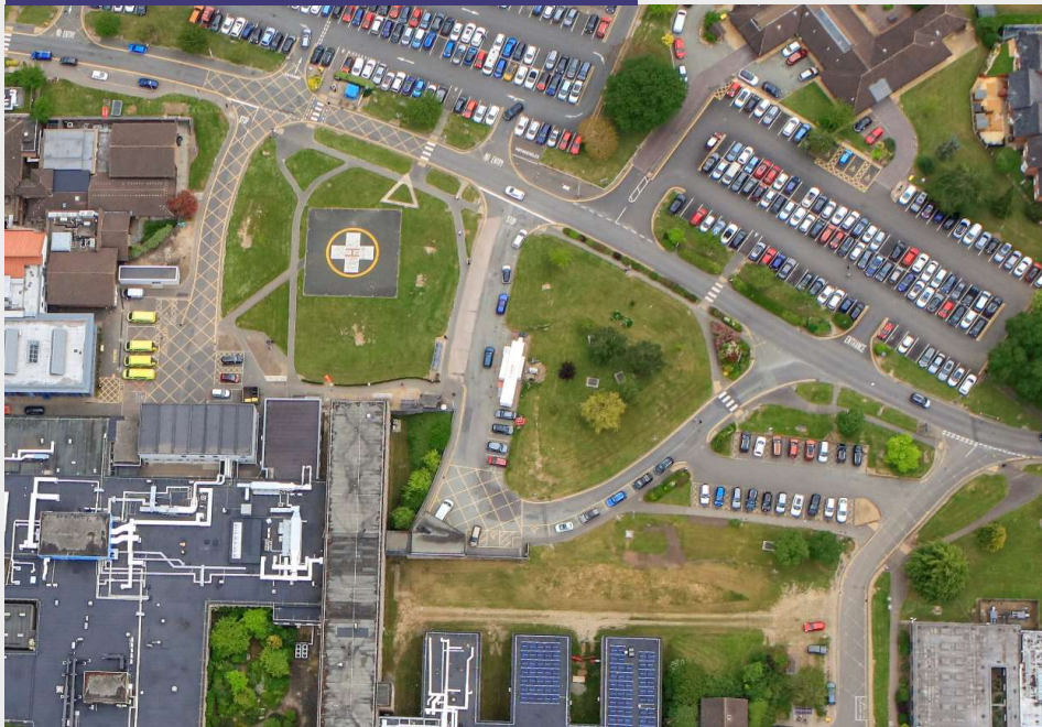
RSH site before works commenced
