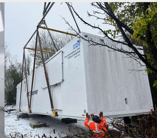
New MRI scanner worth nearly £1.4 million has been lifted into place at the county's first CDC.
